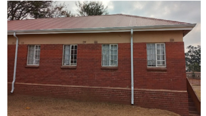
You can be a partner in making this building a comfortable and pretty home for the residents. Call Khantsi @ 017 826 1204.
